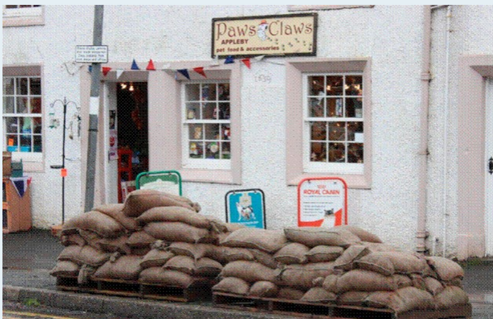
Figure 2: A business in Appleby-in-Westmorland, shortly after one of the frequent floods affecting the area. Note the reliance on sandbags, whose effectiveness is limited (Harries, 2009).
